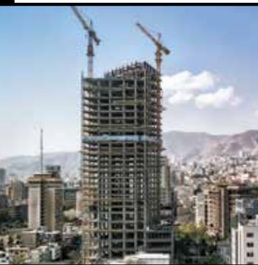
..... Steel framework for the Melal Hotel project
