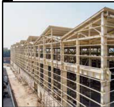
..... Steel Structure Hall of Press Shop-2 for Sanaye Iran Co.
