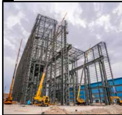
..... Steel framework of the smelting plant of the Sepid Farab Kavir Steel Complex
