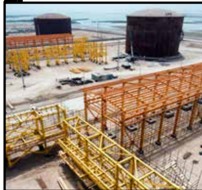
..... Steel structures of the Persian Gulf Bidboland Gas Refining Project
